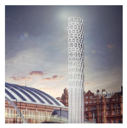
The Tower of Light would be 38.7 metres tall and would be constructed as a vertical single-surface whose strength comes from its form. It would be manufactured from tailored stainless steel sheets which are welded together to create a stiff, strong surface. It would be coated with a matt, pure-white, three-coat paint finish.
